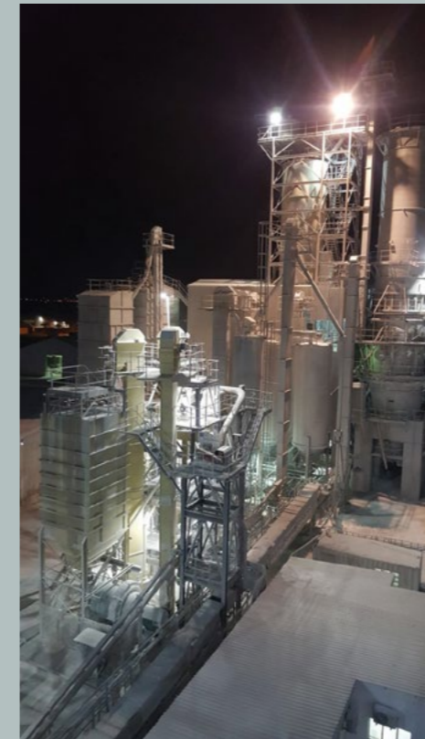
Vredendal Hydrator and OPP Plant at night
