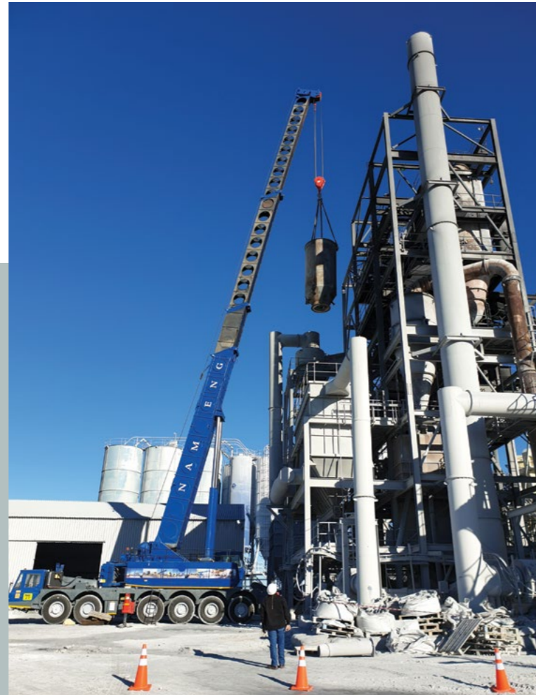
Kiln preheater refractory replacement shutdown July 2019
