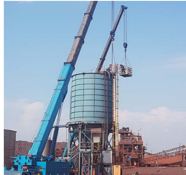
Erection of thickener plant
