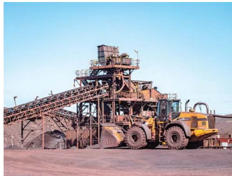
Demaneng reached its design production capacity of 1-million tonnes per annum at the end of February this year
