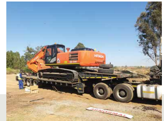
ZX330-10 moving back to site after a quick stop at the ACI Workshop
