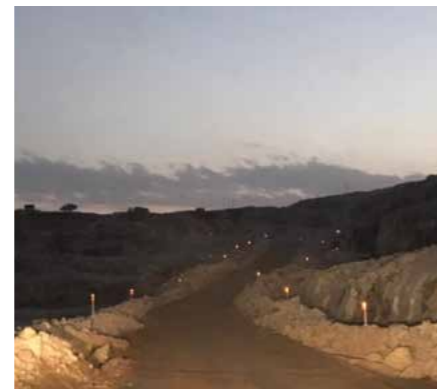
Safety poles indicating the traveling way into and out of the pit
