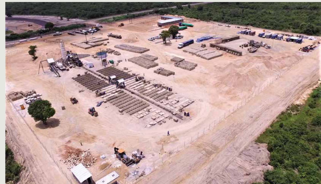
Manguna block yard and staff quarters
