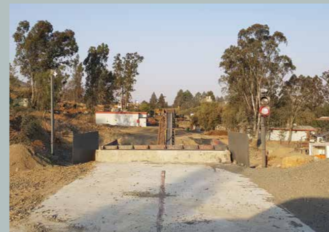
New concrete tipping slab with stopblock
