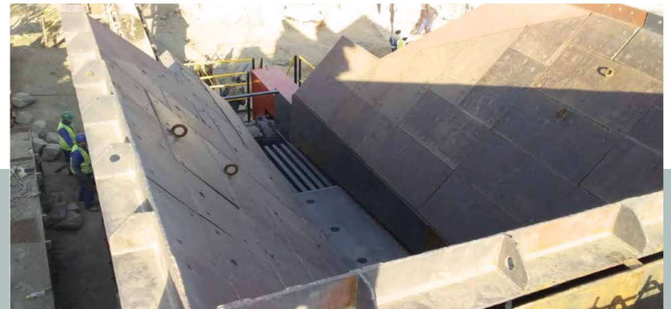
New concrete tipping slab with stopblock
