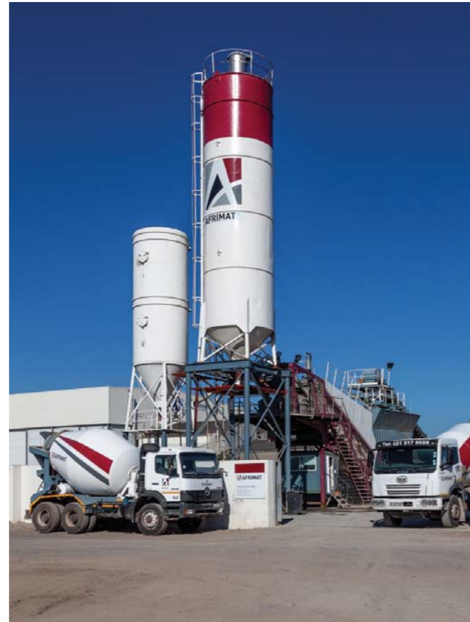
Beautifully branded Readymix silos at the Wetton Plant
