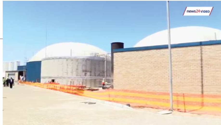
Part of the waste to energy plant in Athlone
