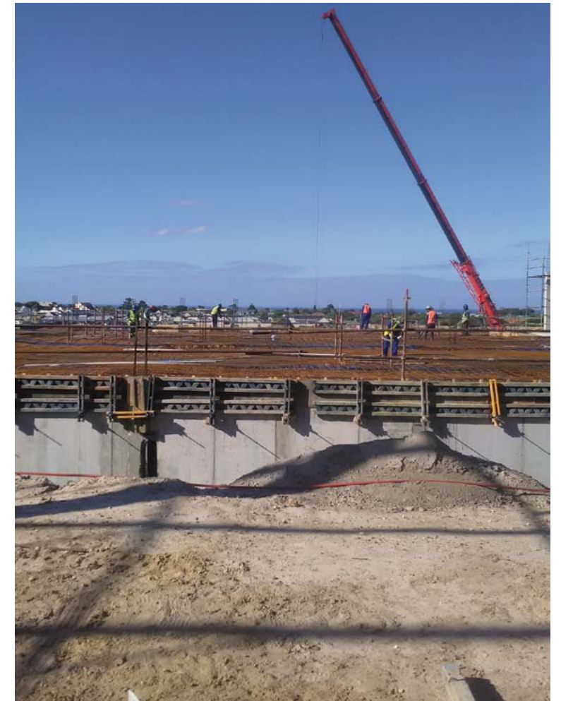
Deck getting prepared for concrete
