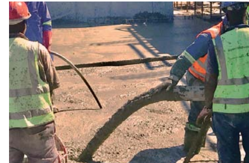
Pumping concrete on surface bed
