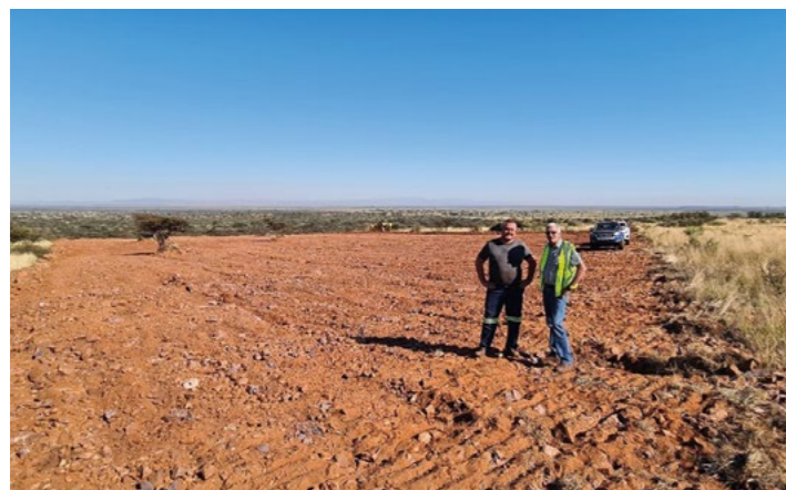
Above: Willie Prins and Attie Delpont at the first groundworks on Jenkins Right (from left): Gerhard Odendaal (MD: Bulk Commodities), Helmut Pool (Independent Non-Executive Director) and Andries van Heerden (CEO) at the iron-ore outcrop on Jenkins before the miners arrived
