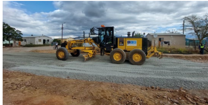
Above: Preparing the road for laying of bricks
