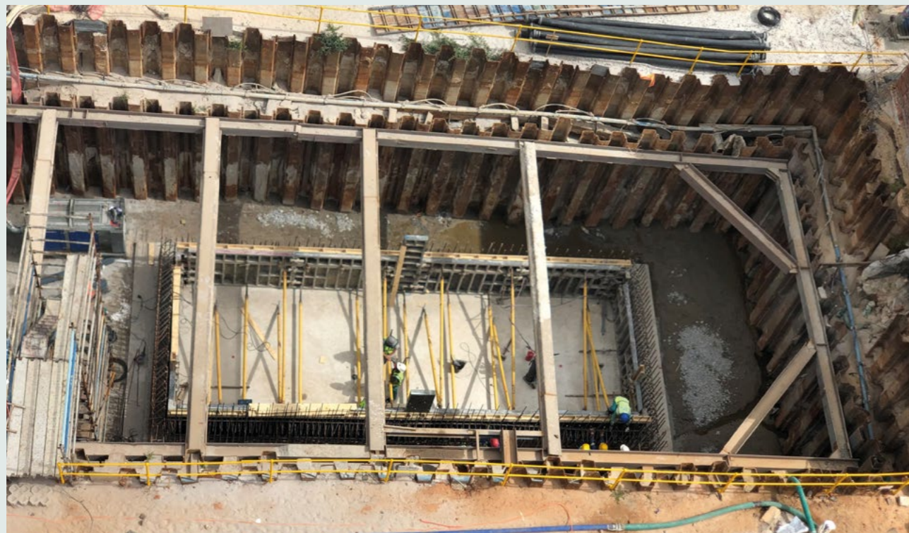
Construction of the Retreat lower lift sewer station
