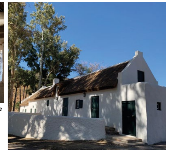
CLC building and plaster lime was used for Wupperthal's restoration project
