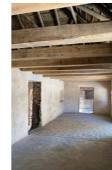
CLC building and plaster lime was used for Wupperthal's restoration project
