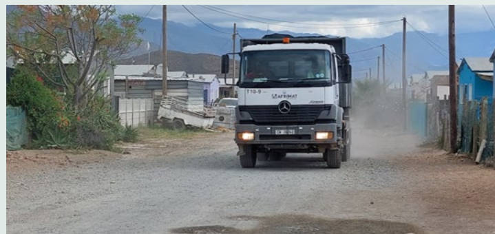
Above: Delivery of aggregates. Right: Laying of interlock pavers
