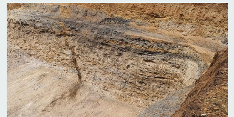
The new highwall ready for portal excavation
