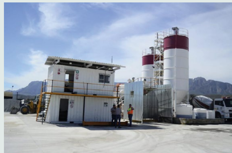
Readymix plant at Boublok
