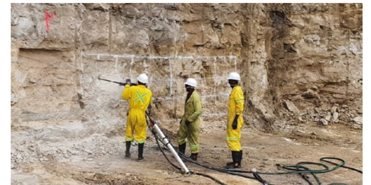
Commencing with drilling for the first portal
