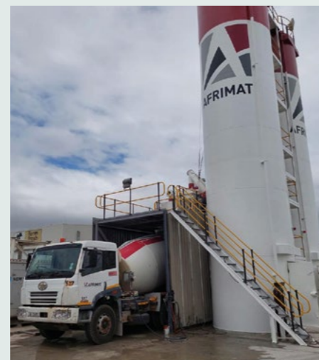
Wetton Readymix plant
