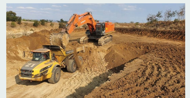
Starting the new boxcut
