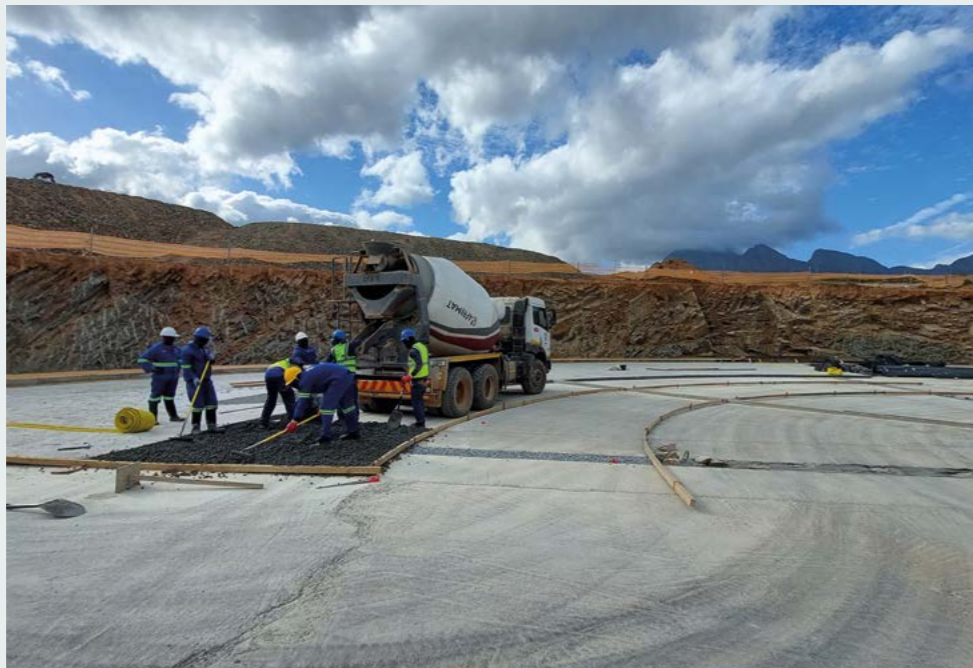
Afrimat Worcester Readymix is supplying concrete for the Worcester Reservoir
