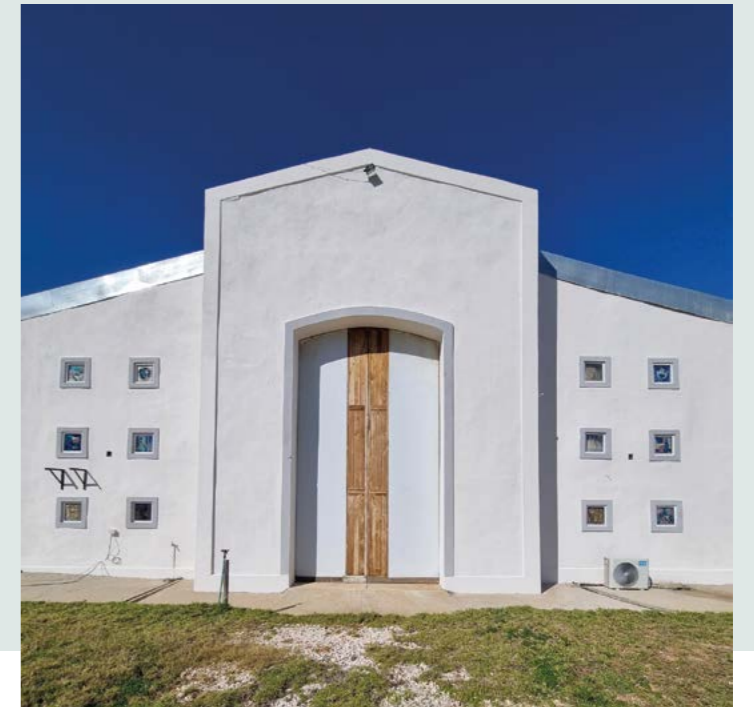
The painting process is complete
