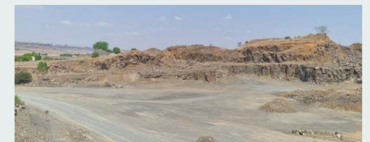
The pit cleaning-up efforts
