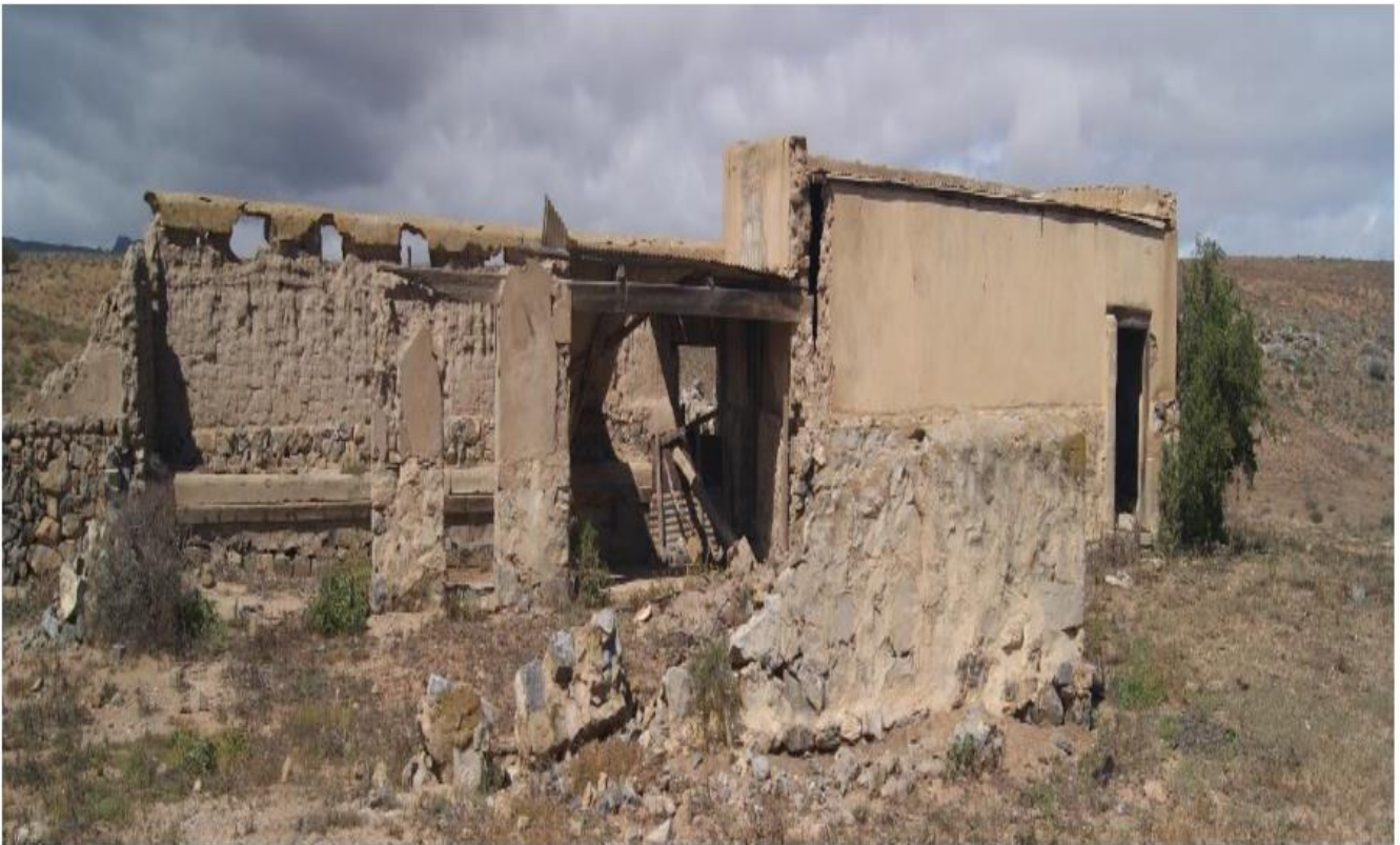
Figure 16: Possible historical structures approximately 200m from the proposed access road route.
