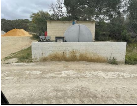
Photo 1: Steel banded diesel tank with a carrying capacity of 110%
