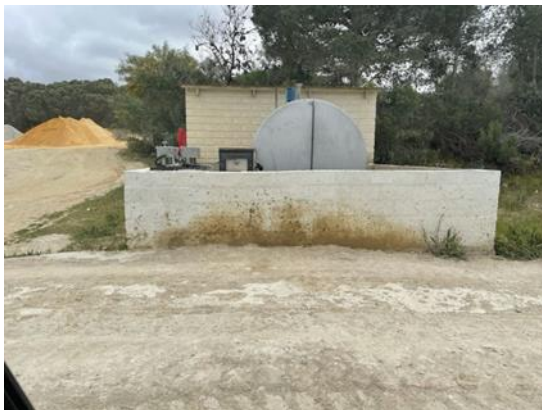
Photo 7: Steel bunded diesel tank with a carrying capacity of 110%
