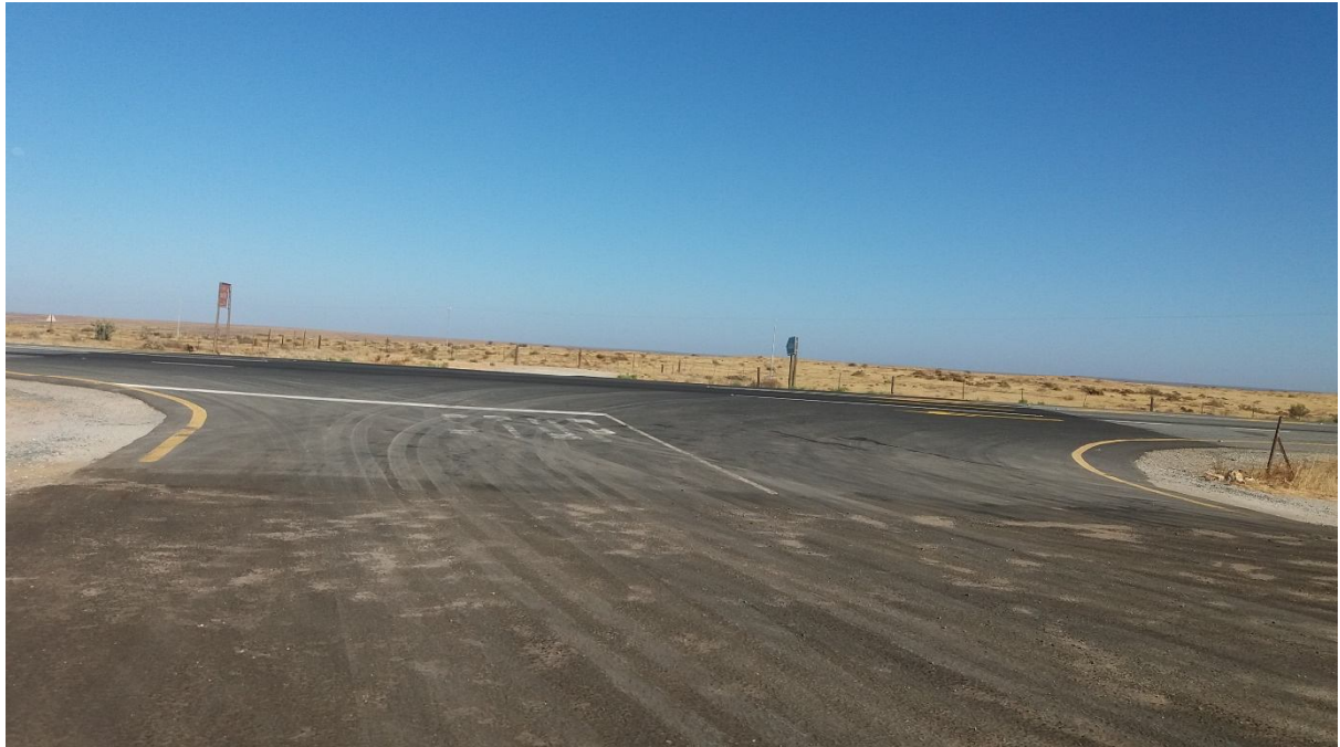
Tarred access road to the site from N7
