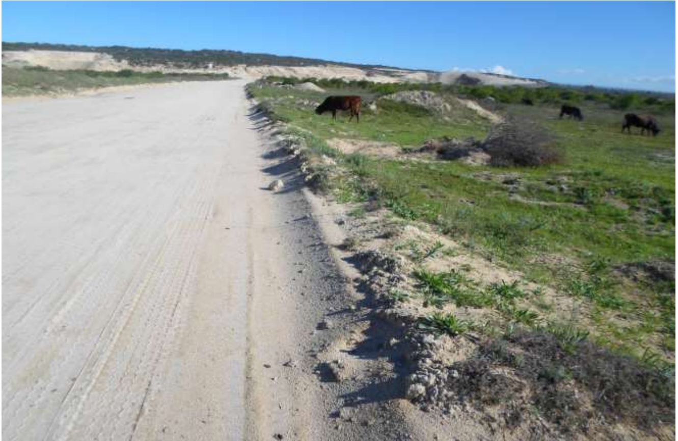
Plate 1: Photo 1: View of an existing road cutting through the proposed development site (Photograph © by Author 2021).
