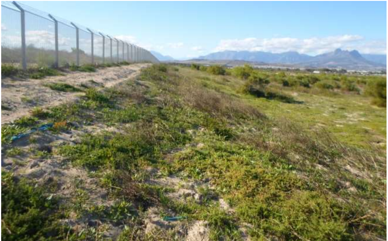
Plate 3: Photo 3: Showing the boundary with the wastewater treatment plant. (Photograph © by Author 2021).
