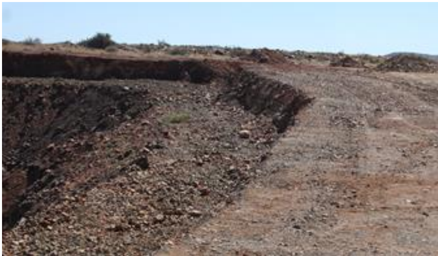
Photo 5: Typical perimeter safety bench during hard-rock quarry rehabilitation
