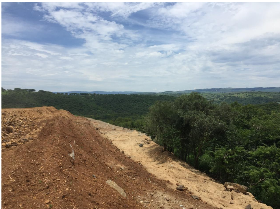
Figure 17: New overburden spoil site (terraced) on northeastern side of mine
