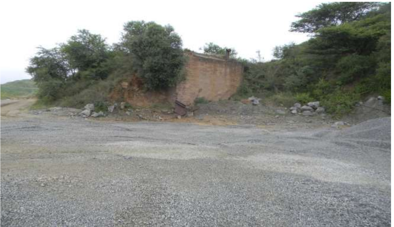
Plate 5: showing the leftover infrastructure from previous mining activities.
