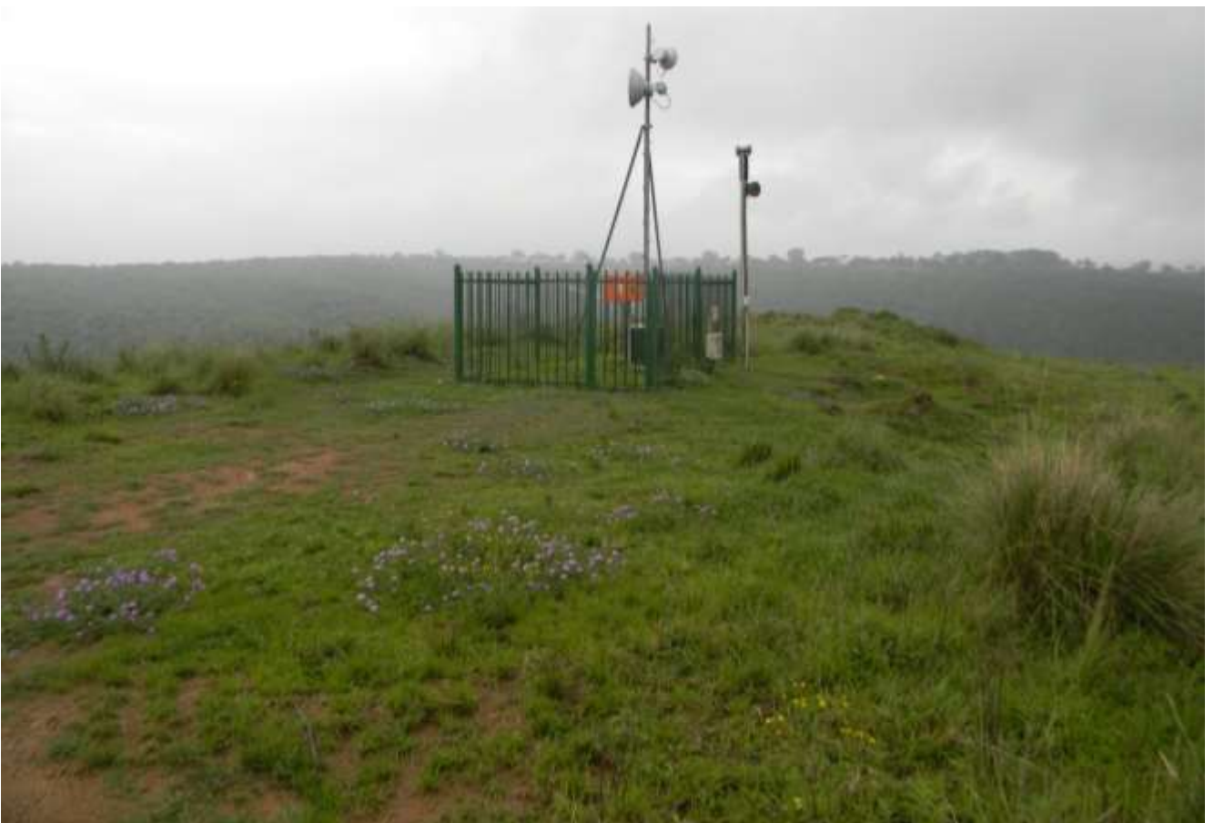
Plate 15: Mine Infrastructure on rehabilitated section within the mining development site
