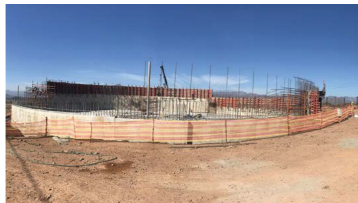
Busy to pumping ringbeam. Below left: Night shift to avoid extreme weather conditions. Below right: Formwork on ringbeam
