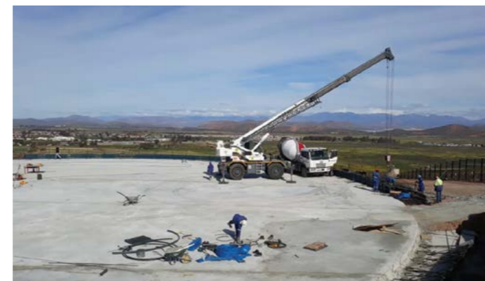
Below: Starting with the ring beam
