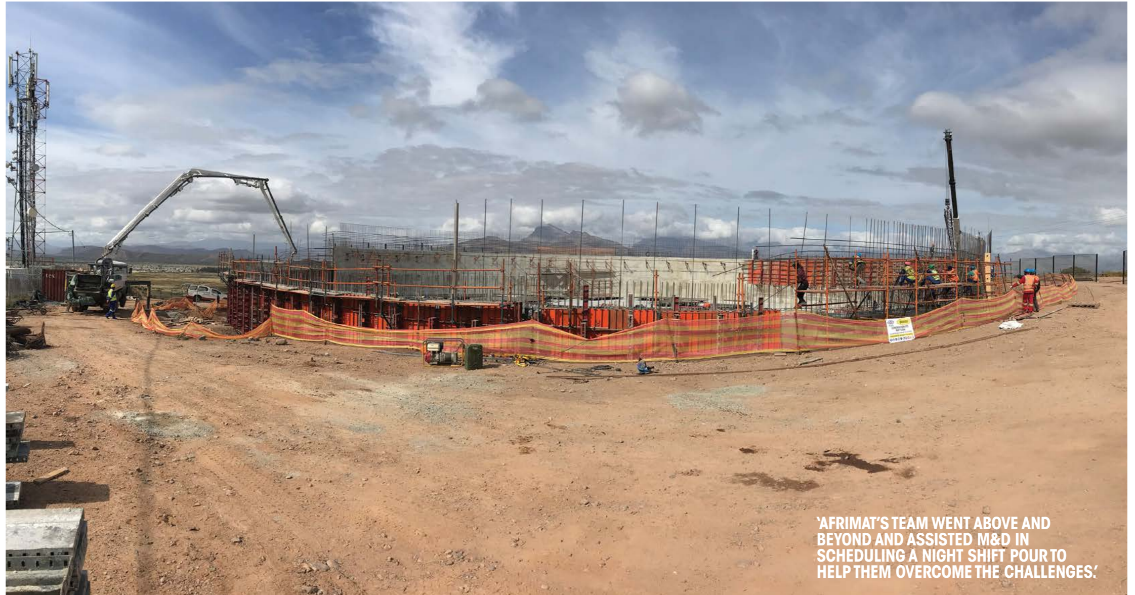
Busy to pumping ringbeam. Below left: Night shift to avoid extreme weather conditions. Below right: Formwork on ringbeam
