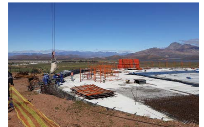
Below: Starting with the ring beam
