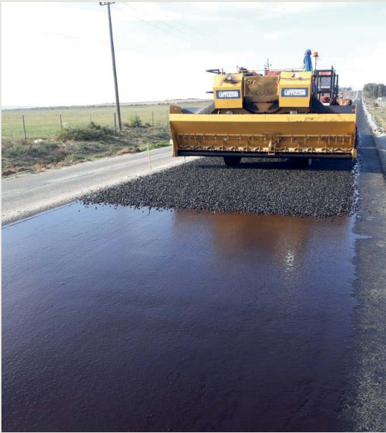
20mm roadstone applied to the surface
