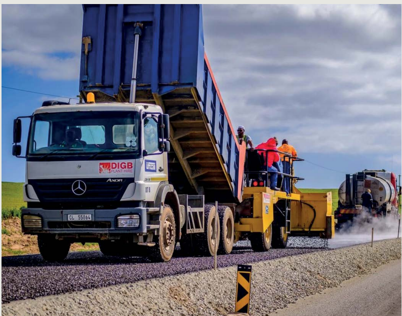
The surfacing operation in progress
