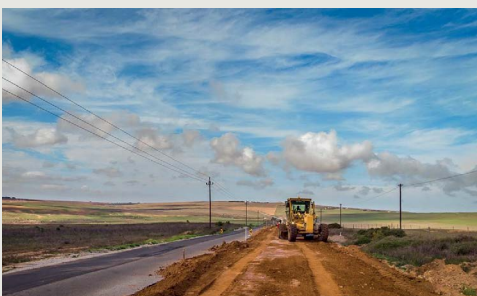
Grading of new section
