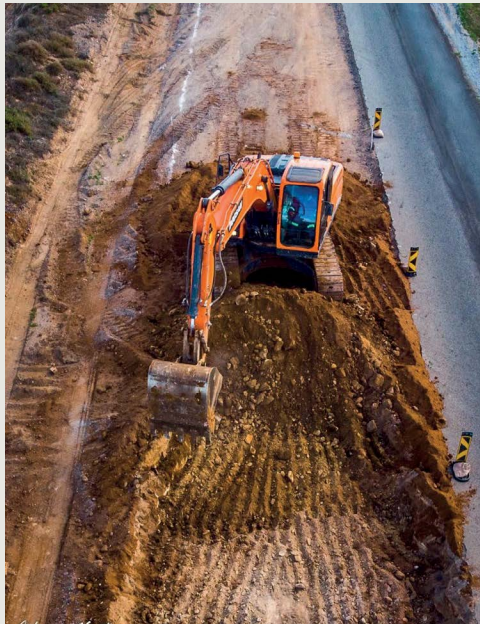
Excavating spoil material
