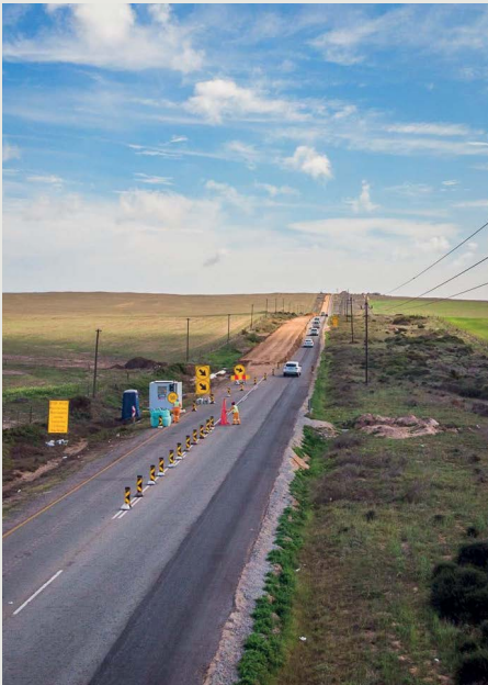
Half-width construction with stop/go operation
