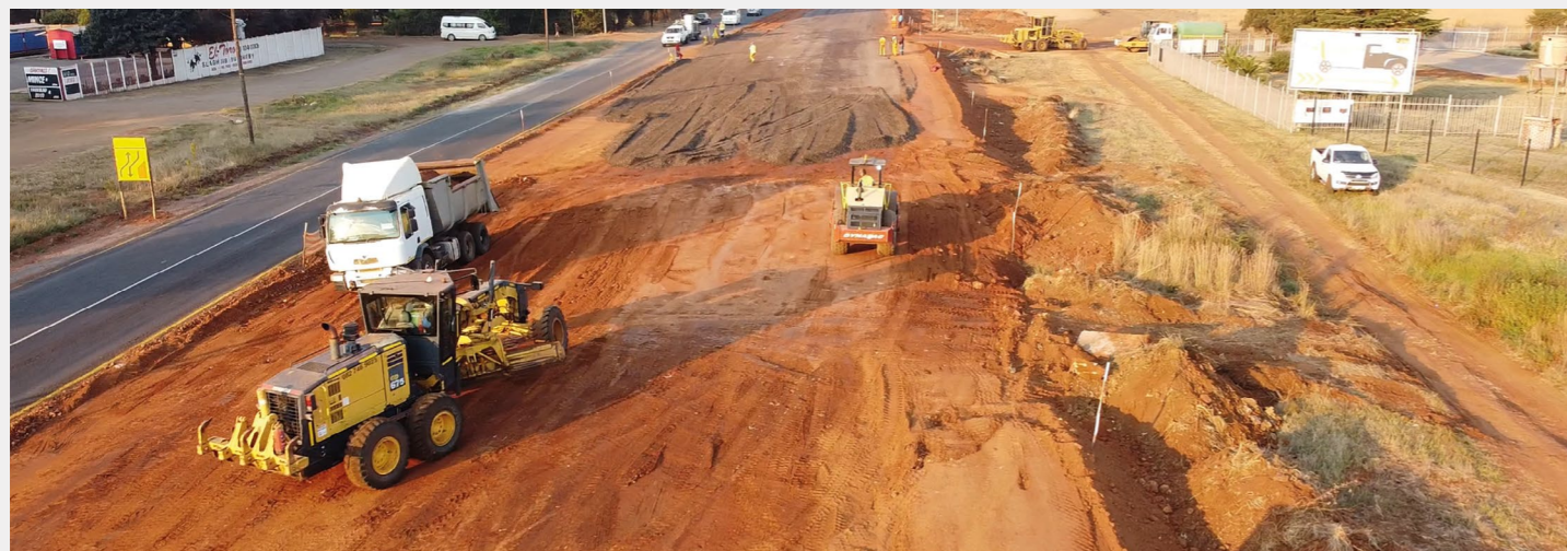
R42 road rehabilitation project
