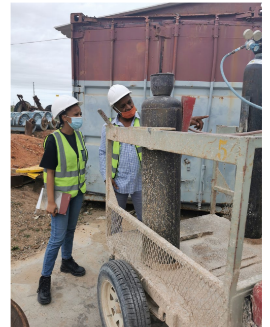
Site safety inspection
