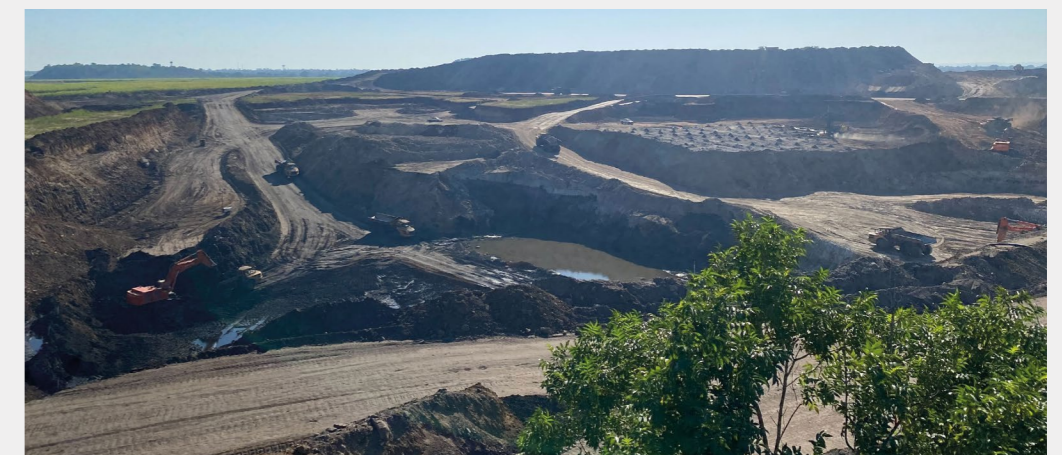
Progress as of mid-May
