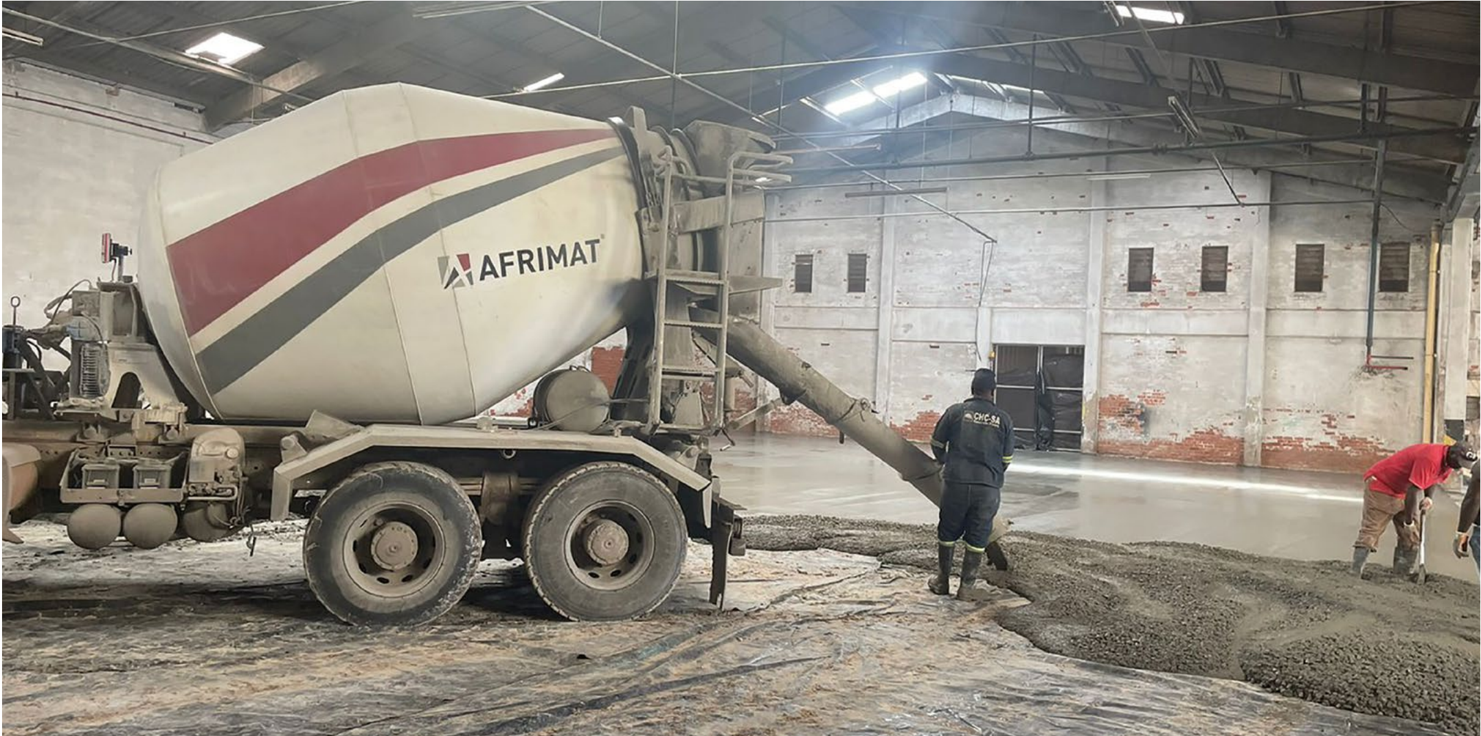
Left and below: Pouring concrete for River Oaks residential development
