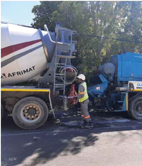
Pumping readymix concrete for the home's three decks
