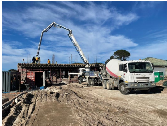
Left and below: Pouring concrete for River Oaks residential development
