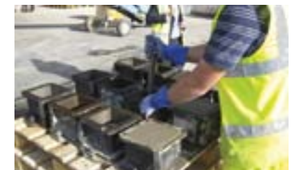
Filling the concrete moulds
