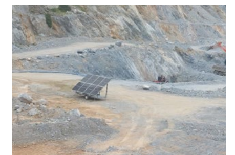
Mobile solar array and float at Langvlei Quarry
