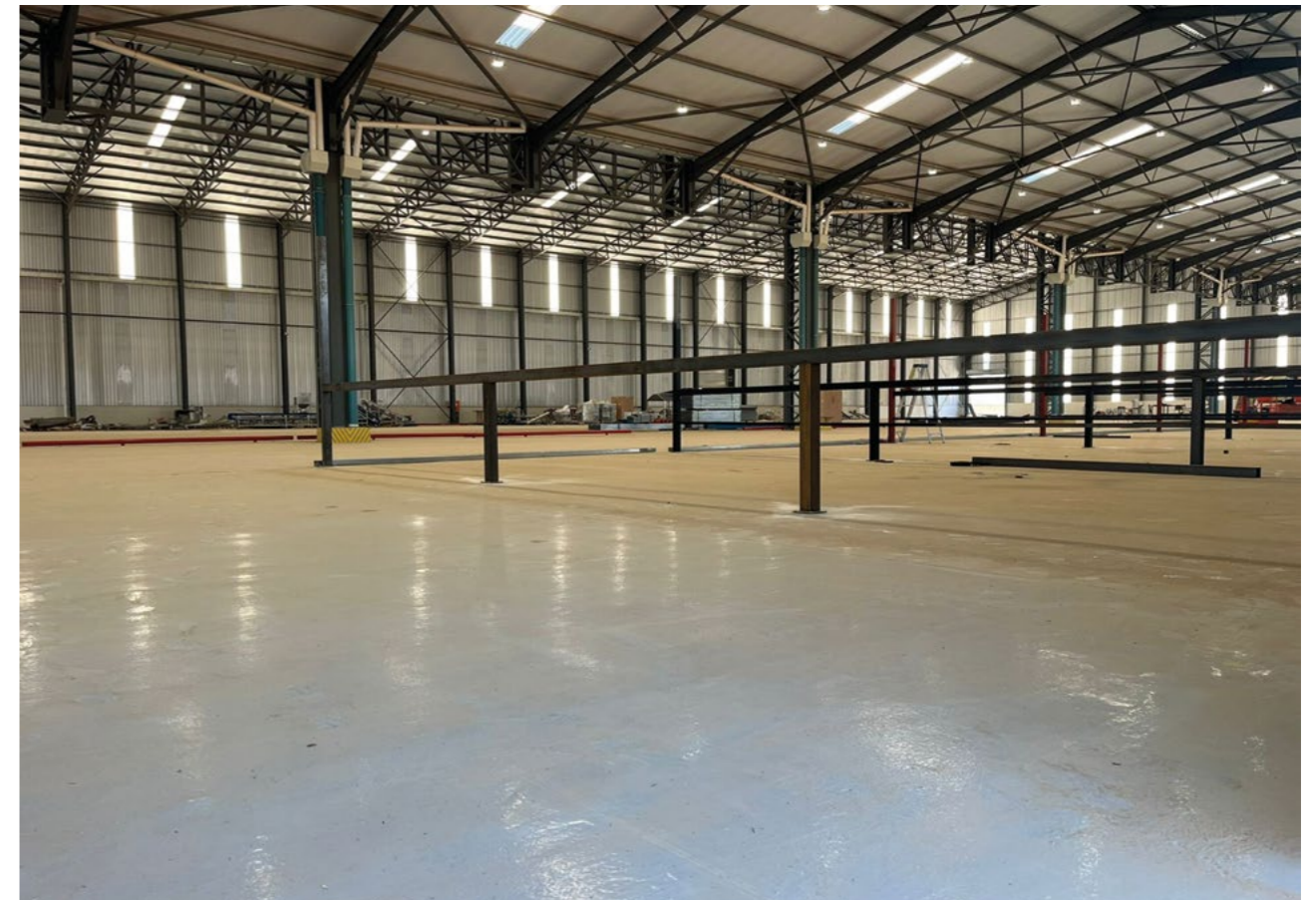
Supplying readymix for the construction project at Truda Foods, Klerksoord
