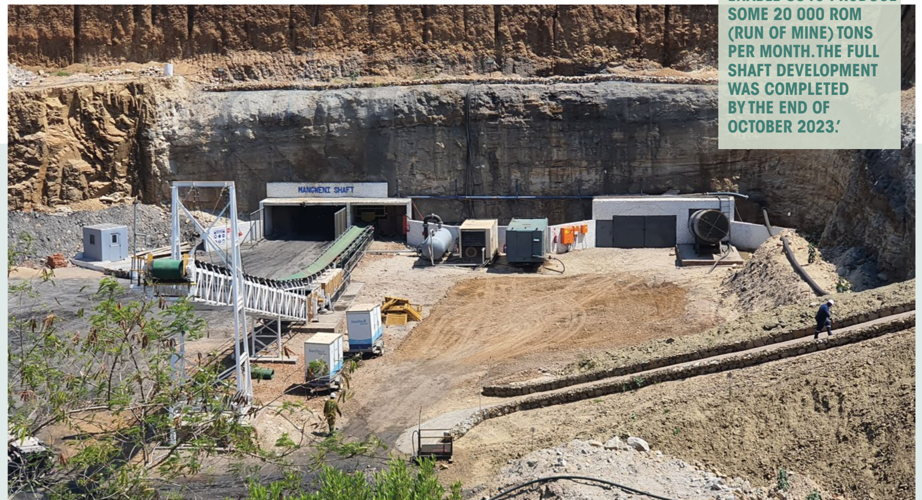
Mangweni underground shaft sinking at Nkomati
