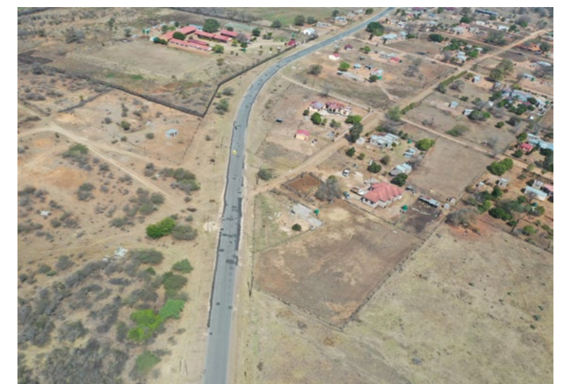
Road repairs in full swing
