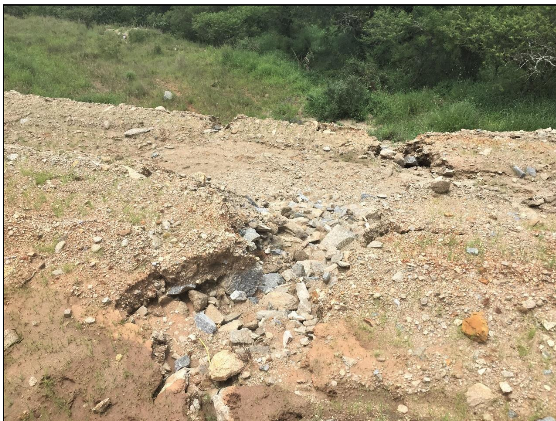
Photo 12 Localised erosion at one of the overburden stockpiles.
