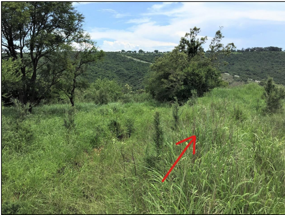
Photo 3 Overgrown stormwater cut-off trench on southern side of mine. The red arrow indicates the direction of flow.
